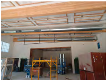
Ductwork installed in the dining area
